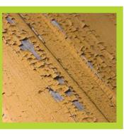
When paint chips off these surfaces, all layers of paint usually come off together. This is a hazard that can cause lead poisoning because the bottom layers of paint may contain lead even if the surface has been repainted with lead-free paint.
